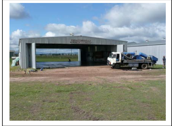
The pump truck cleans up.
