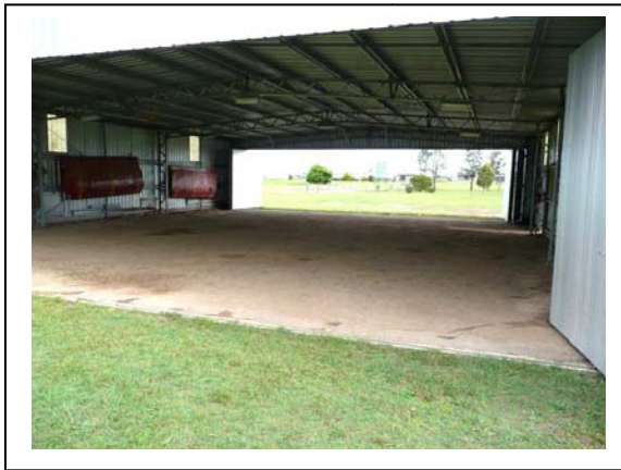
The original carefully rolled and manicured pure dirt floor.
