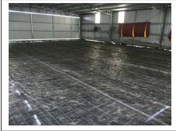
Reinforcing is down, now where's the concrete truck?
