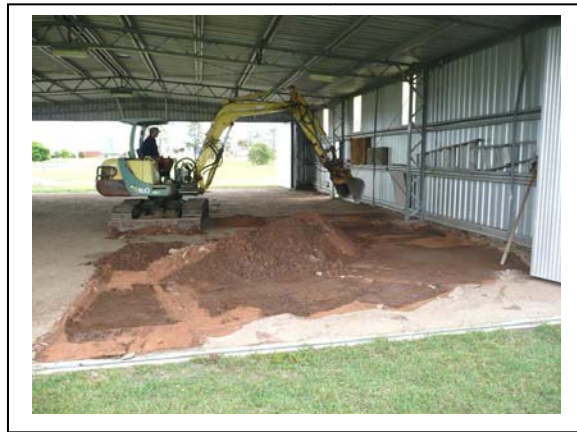
Kevin Werner digging out the bed for the floor reinforcement
