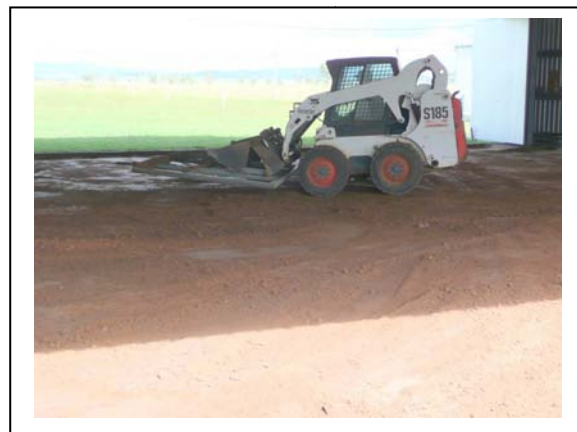
Levelling the excavation.
