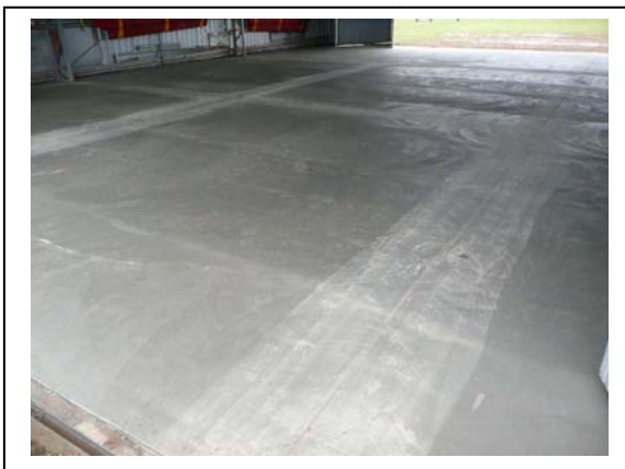
The last job – cutting the stress grooves
